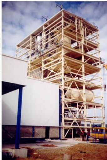
Industrial building - beams in the technological platform
