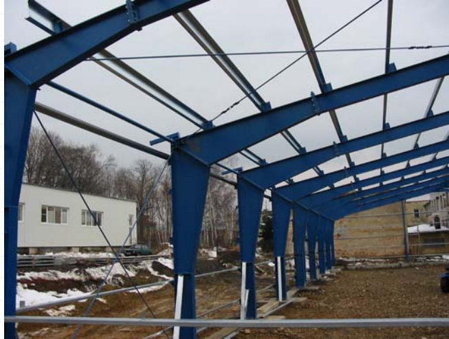
Haunched beams of single-storey building
