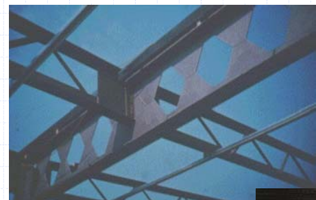
Castellated beam - hexagonal openings
