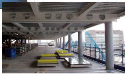
Castellated beam - circular openings
