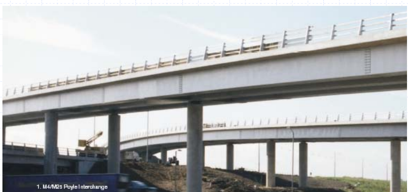
Steel beams of a road bridge
